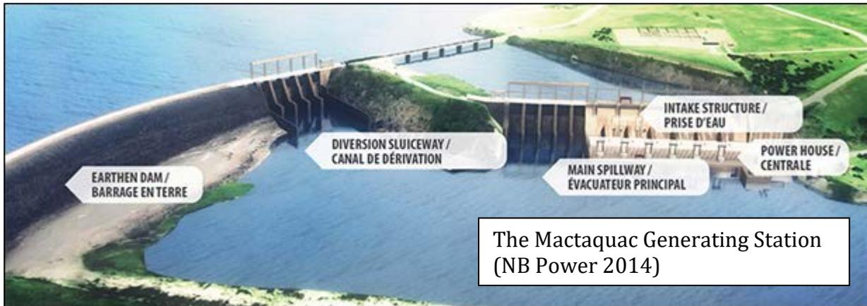
**Figure 2.** Current configuration of the Mactaquac Generating Station.
